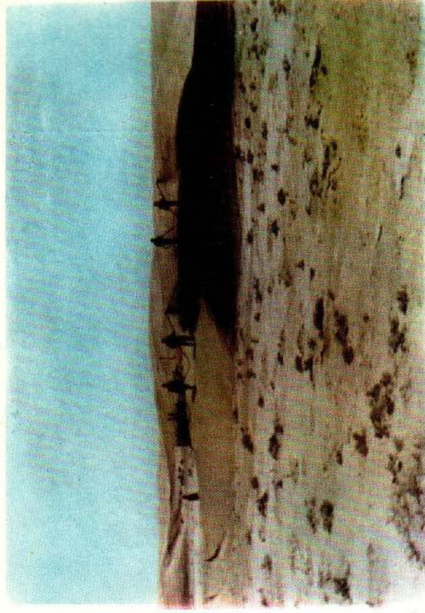
Pouring oil on shifting sands by boom spraying in low sand dune with oil, in Boinzahra area. Trees are held in place while roots firm up.
